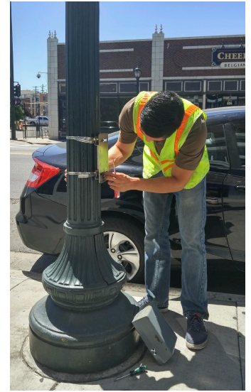
Pedestrian counter being installed at Colfax Ave and Pearl St.
