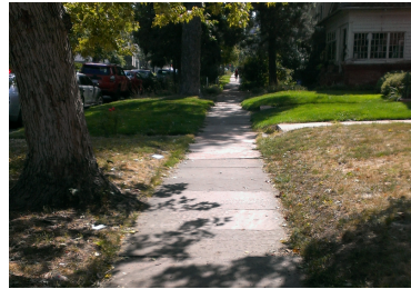
High St between Colfax and 16 th Ave; Less than 5-ft detached; overall quality rating 3 (moderate)
