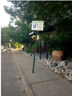
A sign obstructs the sidewalk on Humboldt between Colfax and 14 th Ave.
