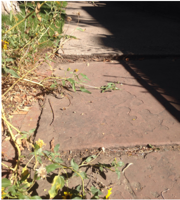
Significantly cracked and uneven sidewalk along Lafayette St between Colfax and 16 th Ave.
