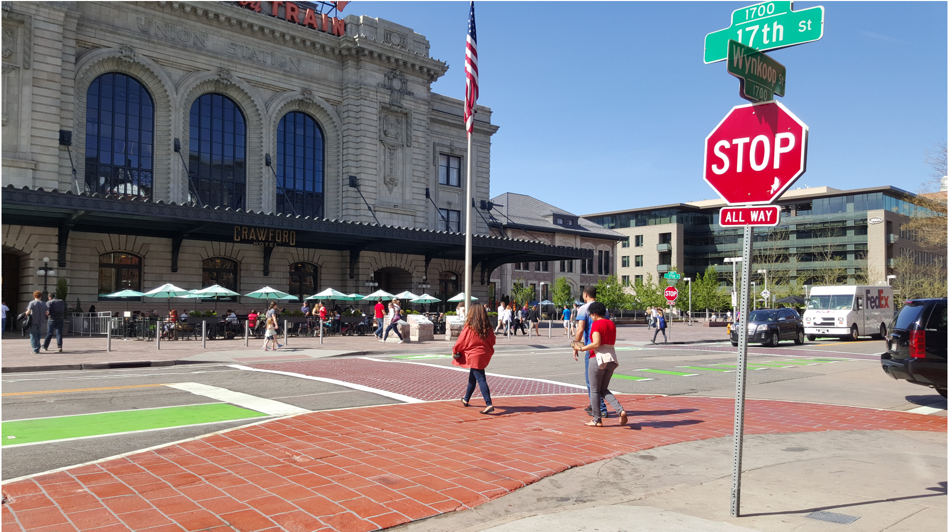
The City and County of Denver used pavement markings to create temporary curb extensions at the intersection of 17 th and Wynkoop. Source: WalkDenver
