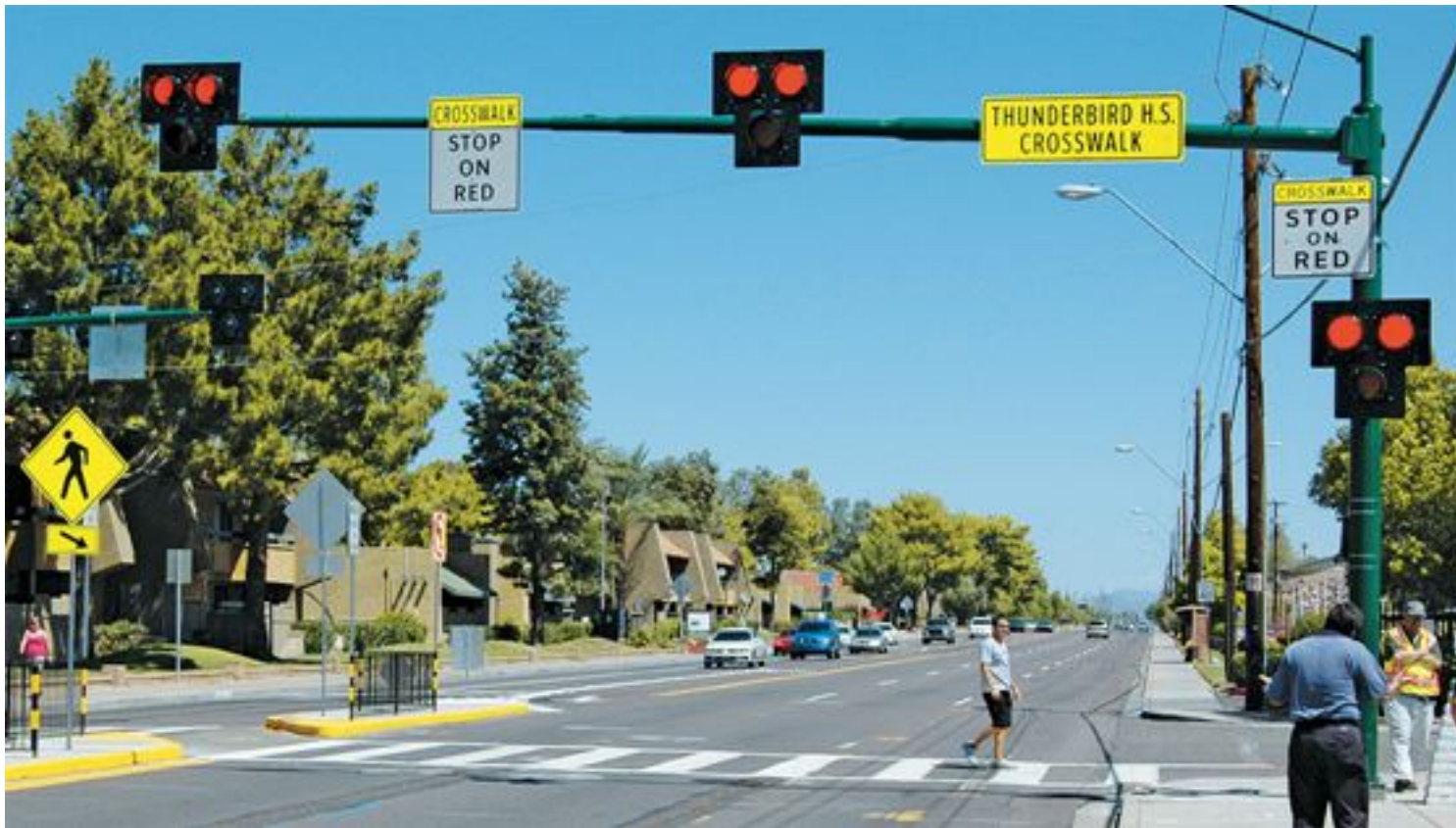
Pedestrian hybrid beacon. Source: Federal Highway Administration.
