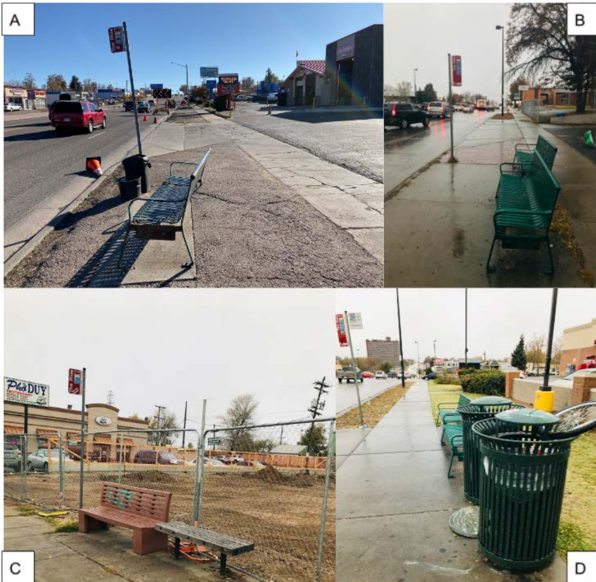
Exhibit 22: Missing Transit/Pedestrian Infrastructure Gaps
