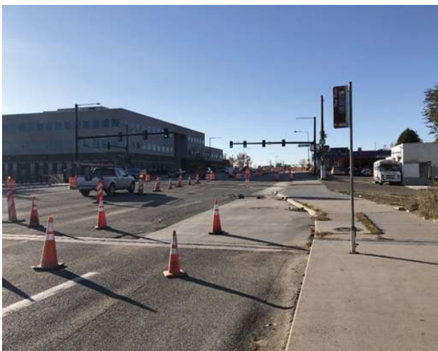
Figure B-3, Bus Stop 13701: Federal Boulevard & West Holden Place
