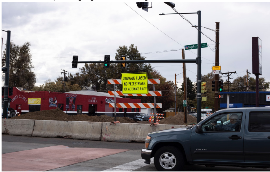
Exhibit 1: An example of ongoing construction along Federal Boulevard
