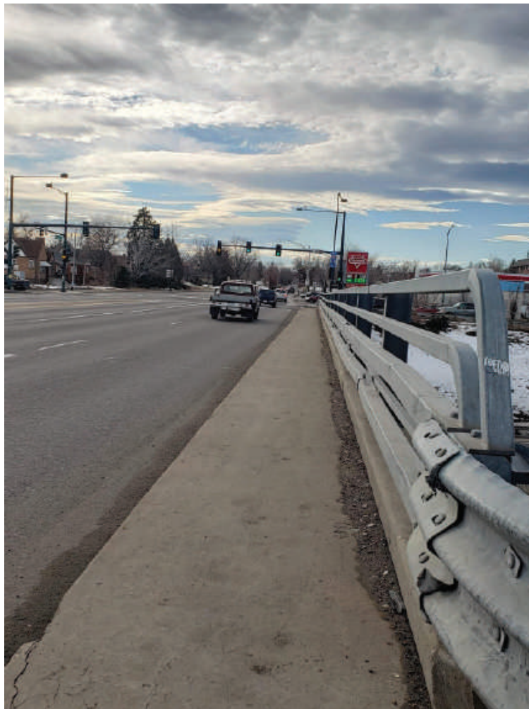
Figure 20: Sidewalk on I-70 Bridge
