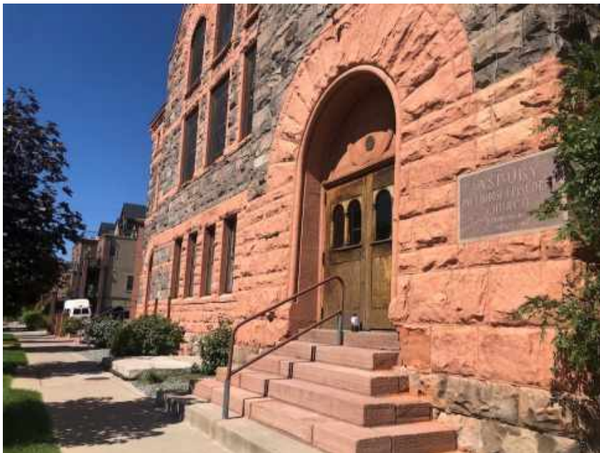
Photo 2: The Denver Dream Center. West 30th Avenue, looking North
