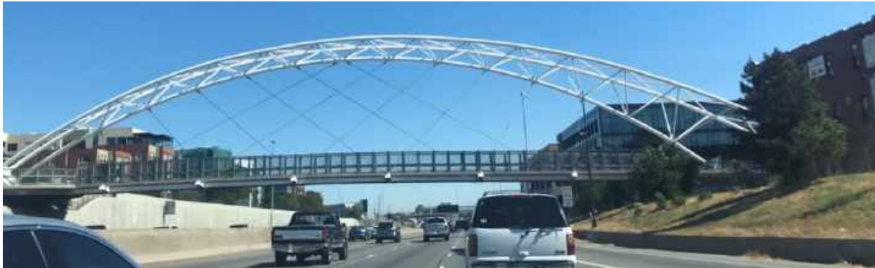
Photo 1: Highland Bridge at Interstate 25 and 15th Street, looking North
