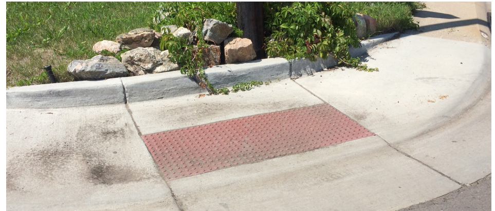
75% of intersections have curb ramps.
