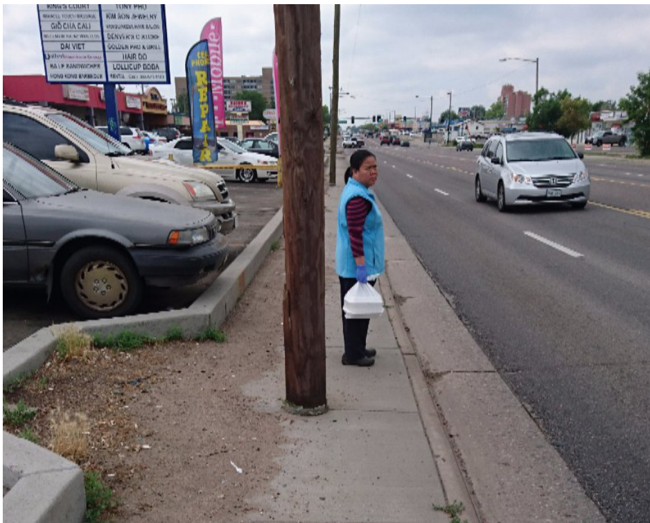
A utility pole obstructs the sidewalk on S. Federal Blvd.
