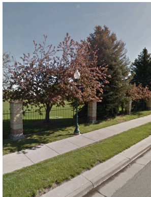
50 th Avenue at Regis University; detached 5-foot sidewalk; overall quality rating 5 (high)
