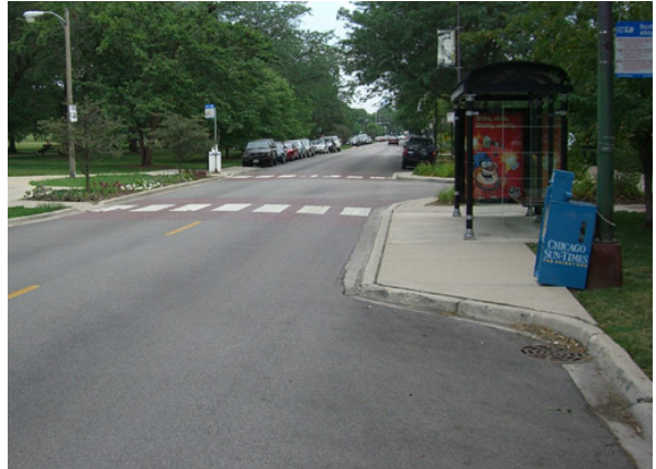
Bulb outs extend the sidewalk and shorten pedestrian crossing distances at intersections.
