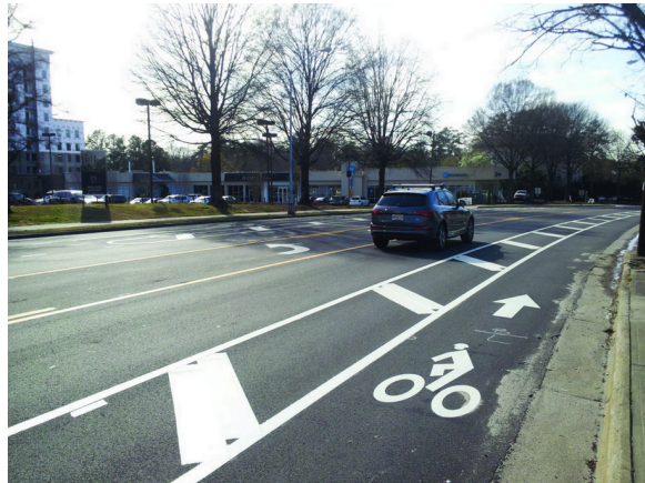
50 th Avenue/Regis Boulevard could be reduced to one lane in each direction by adding a buffered bike lane like this one. Image source: NACTO Urban Street Design Guide.
