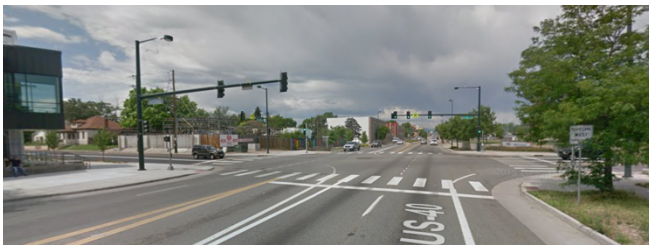
Colfax and Irving existing condition
