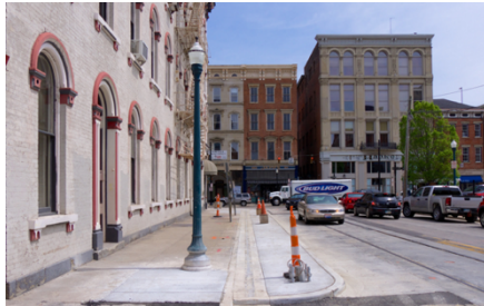
Sidewalk expansion under construction in Cincinnati
